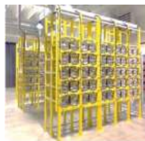
2.5 MW, 100kV HVPS operational at LEHIPA facility, BARC
