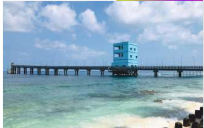
Low Temperature Thermal Desalination (LTTD) plant at Kadamat Island of UT Lakshadweep
