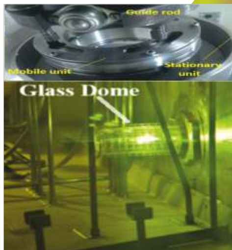
Remotely Operated Self-Locking Fixture installed inside hot cell of wall thickness 1.8 meter
